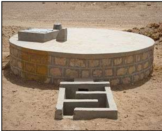
Tanka with artificial catchment and silt trap
