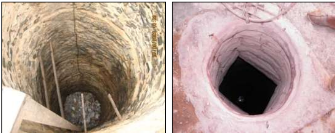
Dug well in hard rock
