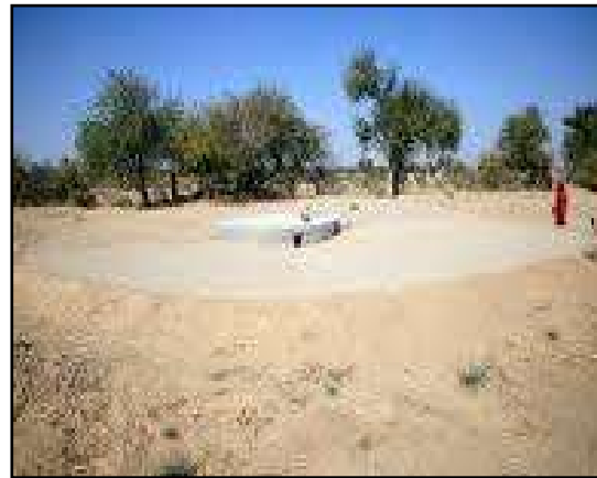
Tanka with artificial catchment and silt trap
